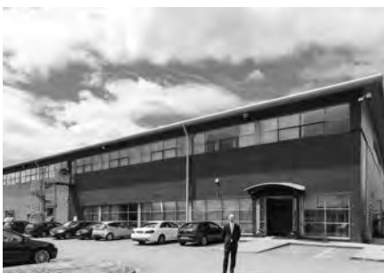
THE 55,000 SQFT RAINHAM FACILITY
